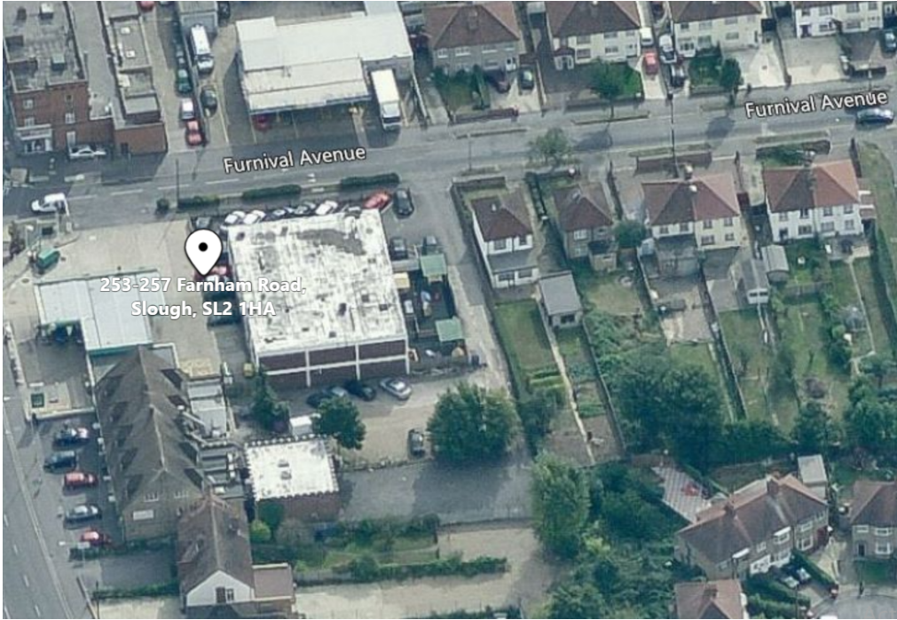
Aerial view from north of existing building
